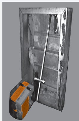
Solution: Belimo FSTF with linkage
